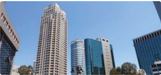
Air conditioning control system – administrative center Ramat Gan – Tel Aviv, Israel
