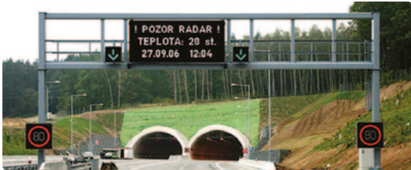
Highway tunnel Valik control Czech Republic
