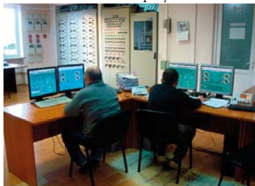
Image: Dispatching room with 2 screens, switchboard with control system Tecomat TC700 from our company Teco a.s.
