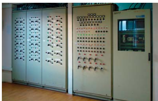
Image: Typical configuration of 2 switchboards for 4 tanks and relevant group of automatically controlled valves.
