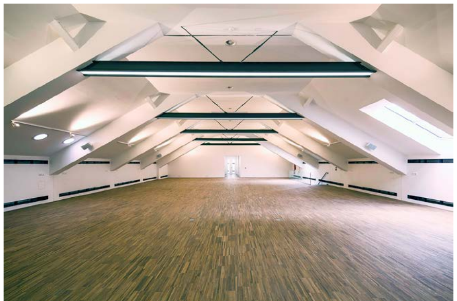
The training hall is the largest room in the building. The lighting system is installed in the roof truss supporting structure.
