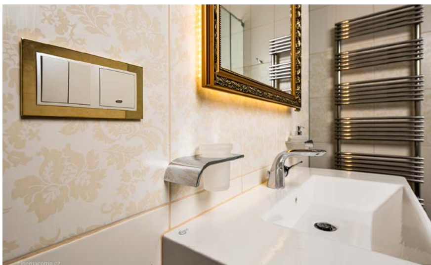
Wall-mounted controllers in the bathroom are also equipped with thermal sensors and control both the mirror illumination as well as the heating ladder. The apartment is also equipped with larger number of wall outlets, illumination circuits and dimming circuits using RGB LED stripes. Further, the apartment also features floor convectors directly controlled by Foxtrot outputs.
