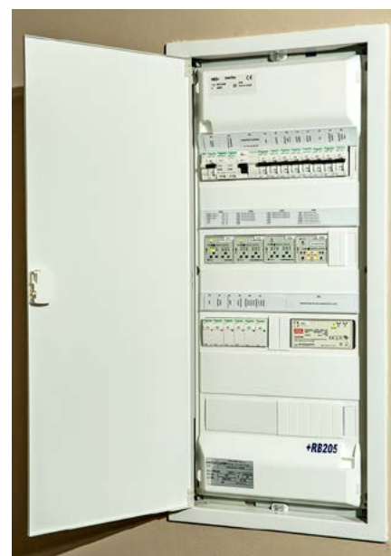
Each hotel room is equipped with a distribution cabinet installed with CFox modules and connected to the central control system Foxtrot via CIB bus.
